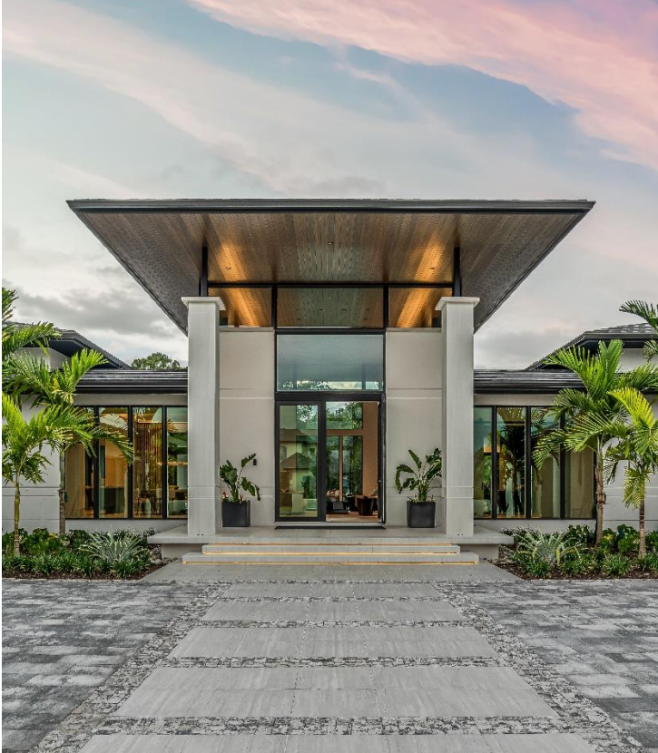
Exaggerated cantilevered roof overhangs with tongue-in-groove ceilings heighten the dramatic contemporary architecture while ingeniously shading large windows for reduced heat gain inside.
